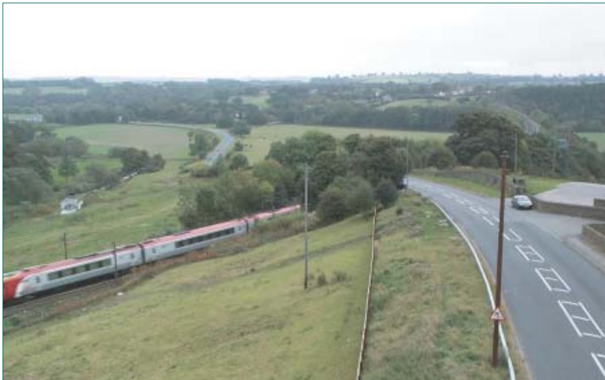
Photo 2b: Bridge site at Browney Lane, County Durham – after treatment
