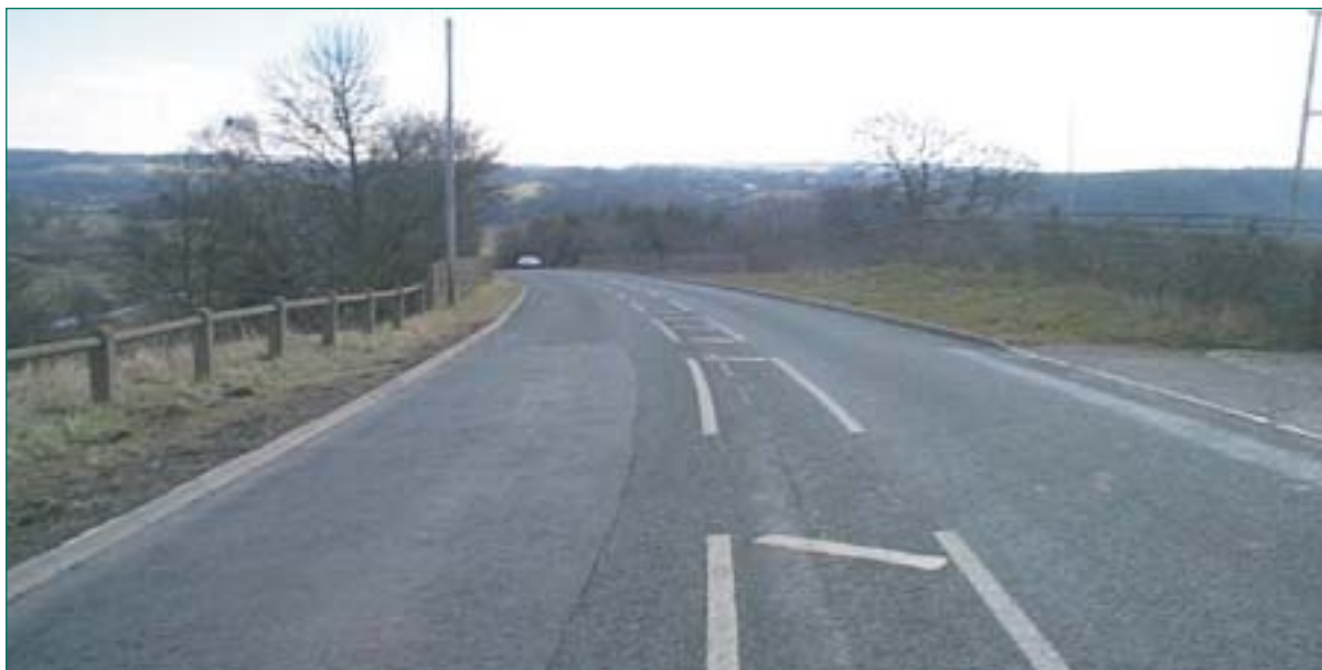
Photo 2a: Bridge site at Browney Lane, County Durham – before treatment
