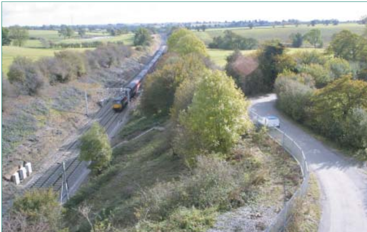
Photo 1b: Parallel site – Ashby St Ledgers, Northamptonshire, mid-installation
